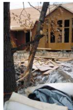
Wounds are often caused by construction activity.
