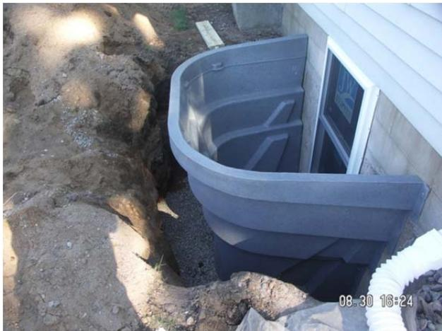
Window well (areaway) with drainage rock under & around it, unit should terminate 8" above grade.
